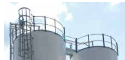
Safety railings and walkways
